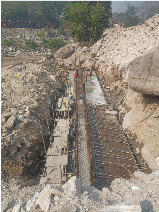
Power House Protection Wall: Floodwall
