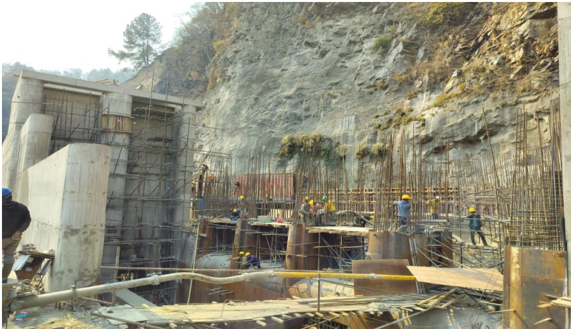
Concrete Works at Intake
