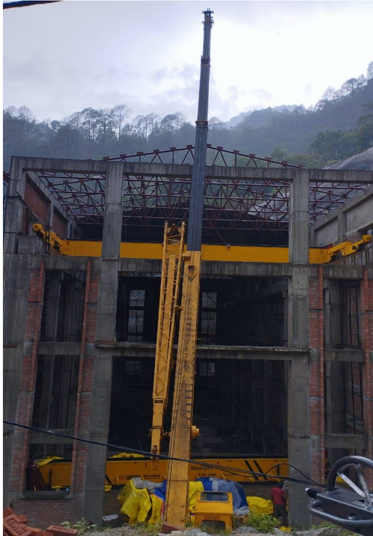
EoT Crane Installation
