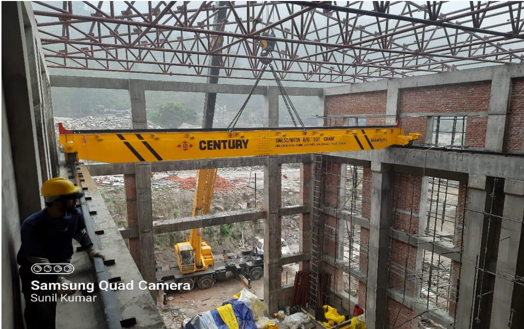
EoT Crane Installation
