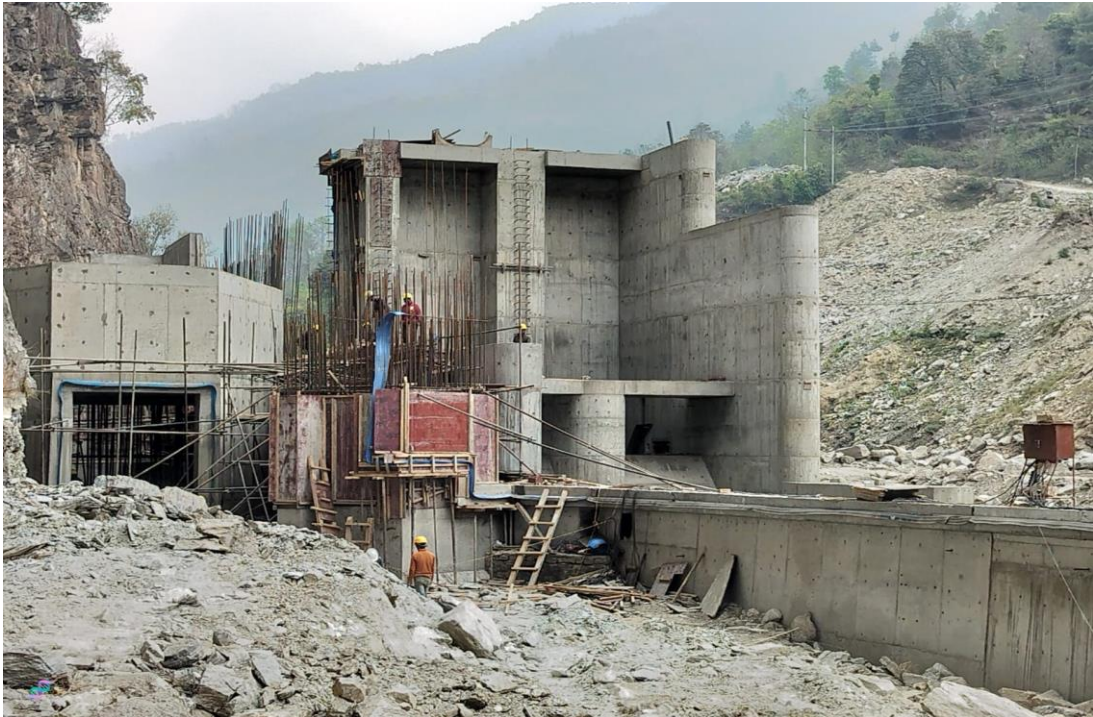
Flushing Chamber Formworks
