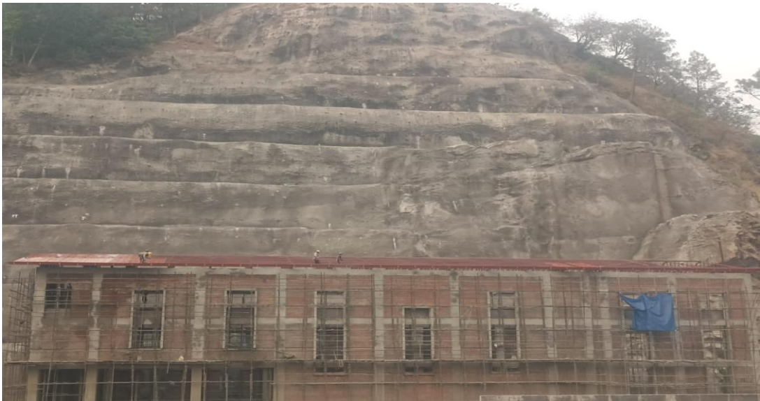
Roof Works at Powerhouse
