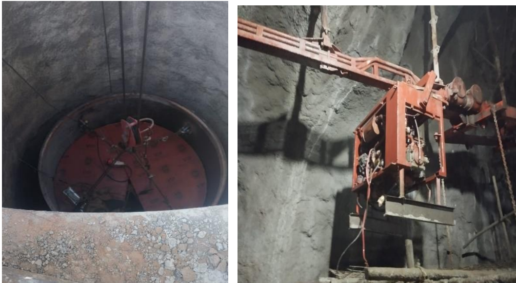
Upper Pressure Tunnel and Vertical Shaft-2 site
