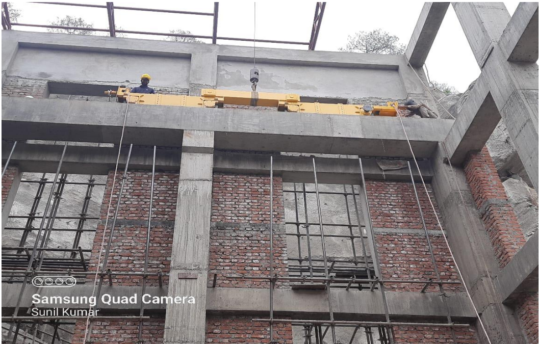
EoT Crane Installation
