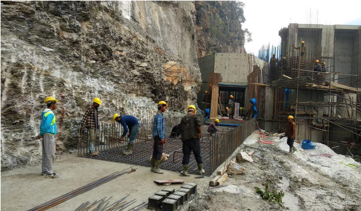
Approach Culvert Rebar Works
