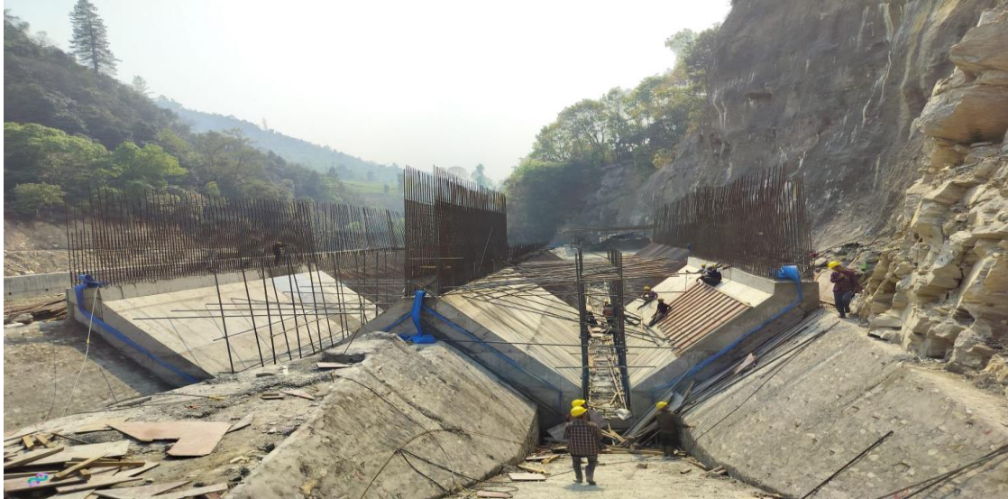
Deshuttering Works at Desander
