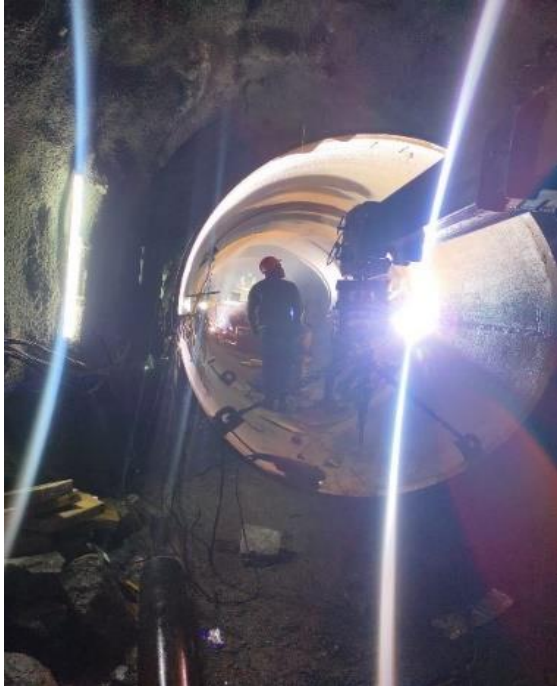
Pipe welding, pipe lowering
