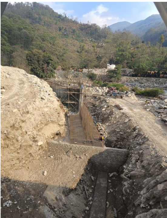
Power House Protection Wall: Floodwall
