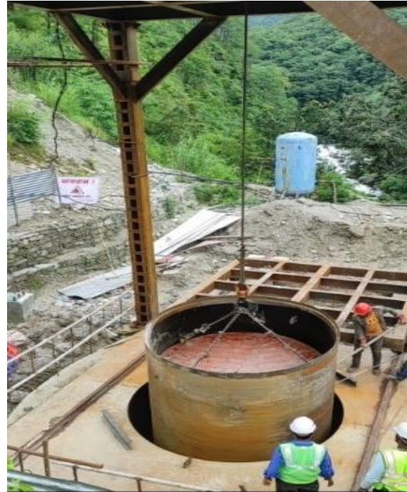
Pipe welding, pipe lowering
