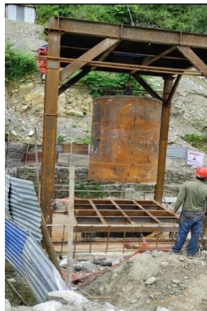
Pipe welding and pipe lowering in VS-2
