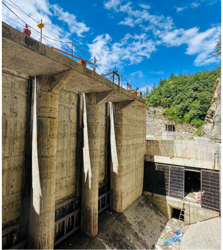
Headworks intake Undersluice area
