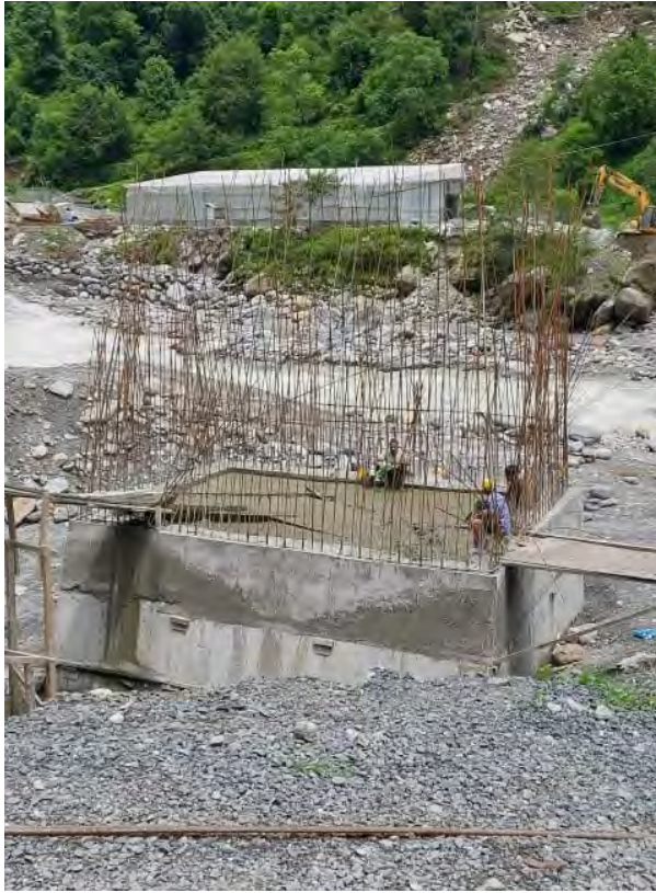
Construction of Powerhouse Access Bailey Bridge.
