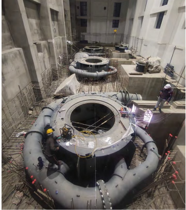
EM Works Erection of Turbine casing and distribution pipes
