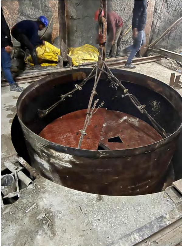
9 HM Works Penstock Pipe Lowering Works in Vs1
