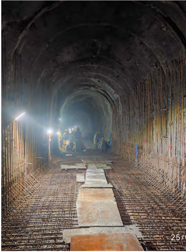
Headrace Tunnel Final Lining Works
