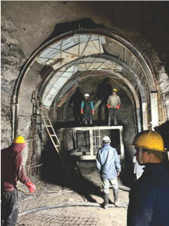
Rib installation in HRT
