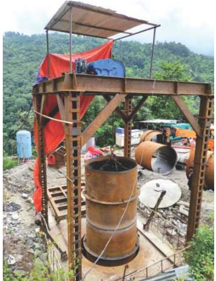
HM work Lowering of Pipe in Vs2
