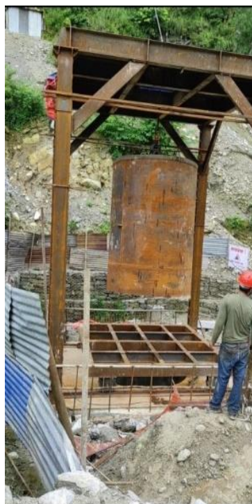
Pipe welding and pipe lowering in VS-2
