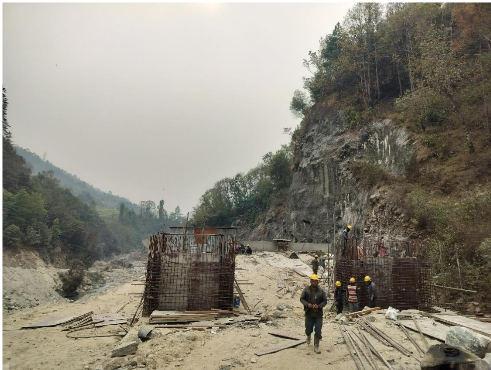
Formworks at Settling Basin Inlet Gate
