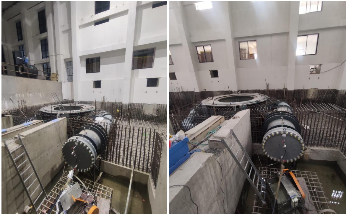
Pressure test on ring line of unit 1 and 2
