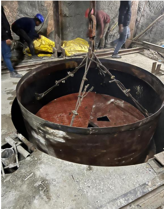
Penstock Pipe Lowering at VS-1
