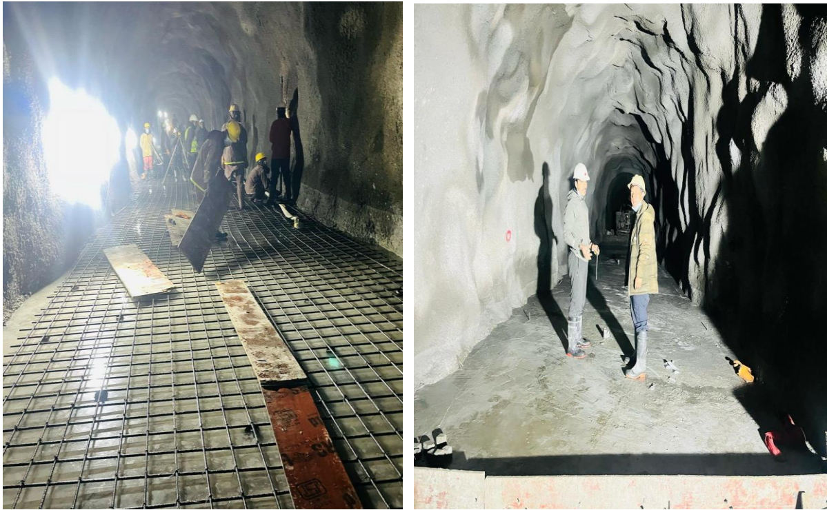
Inlet Lining works
