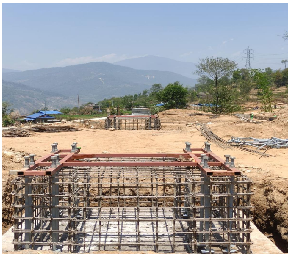
Foundation bolts installation of gantry at LLO
