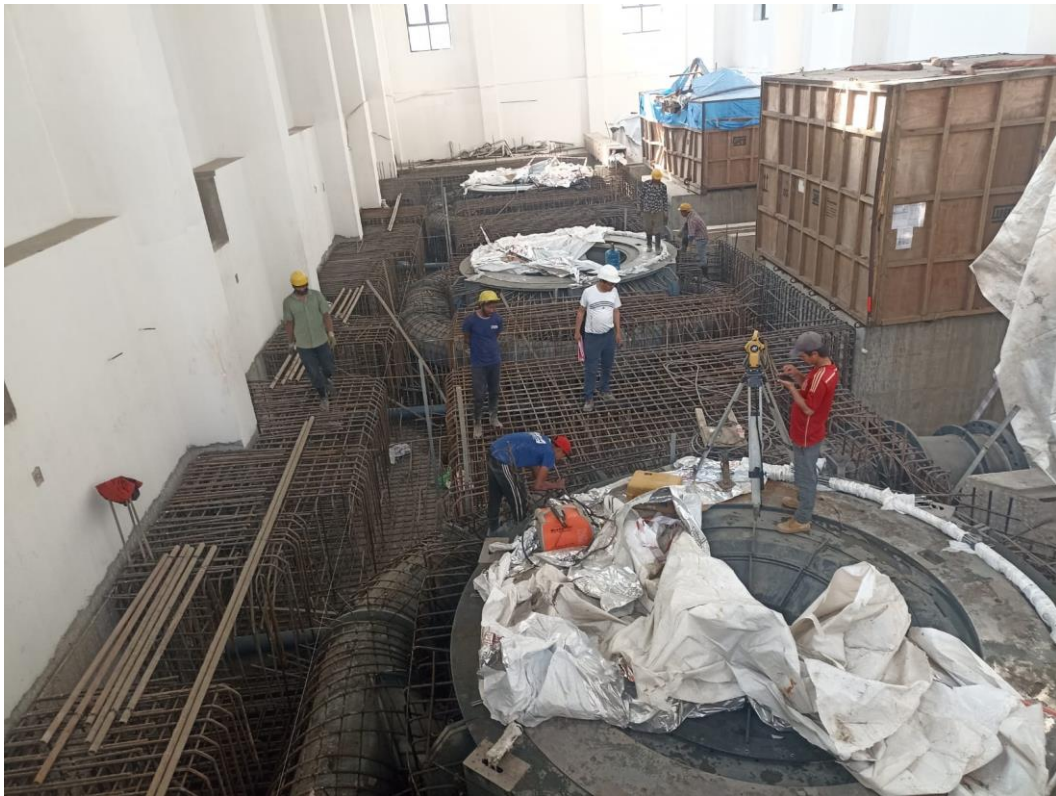
Powerhouse second stage rebar works ongoing
