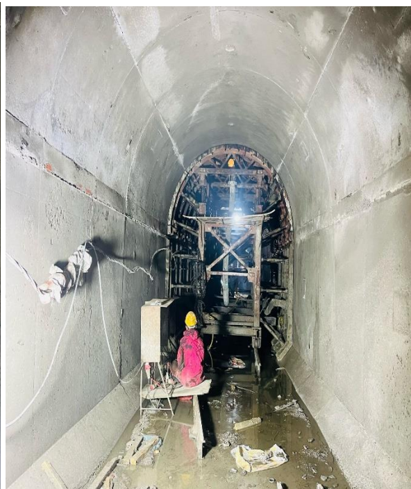
Lining works from Face 2 (Invert, wall and arcs)
