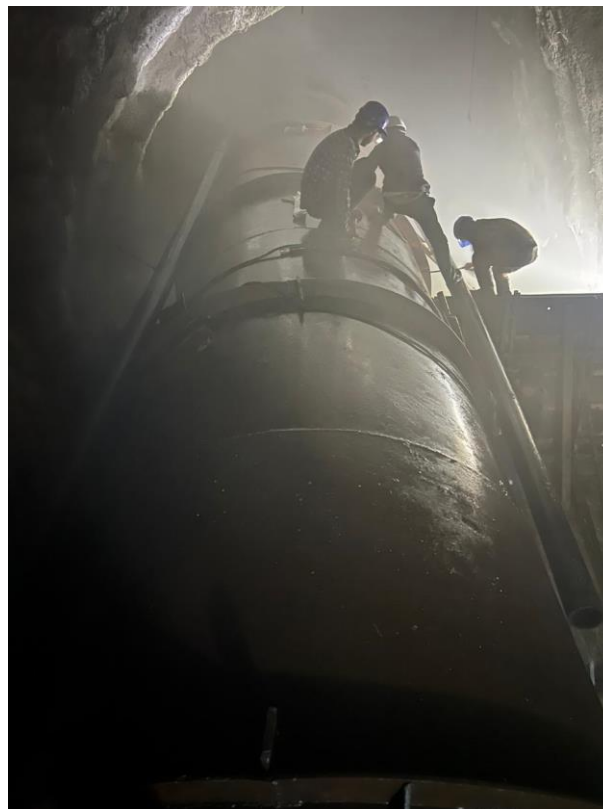
Drainage Pipe Installation at UPT
