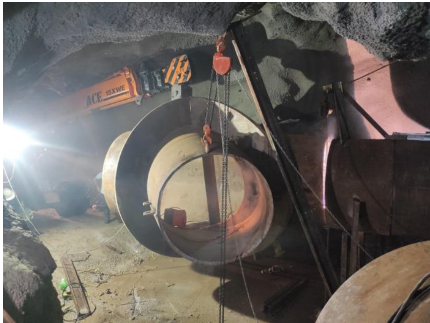
Bifurcation-I Erection Works
