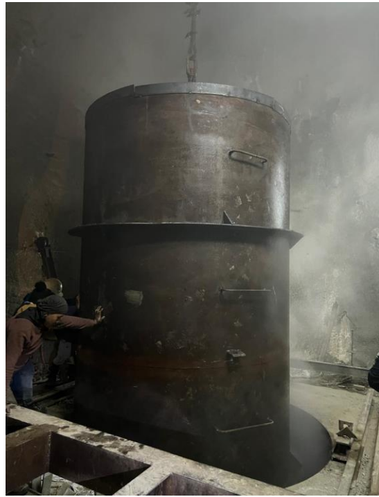
Penstock Pipe Lowering at VS-1
