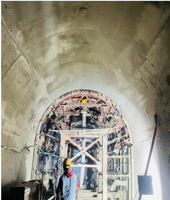
Lining works from Face 2 (Invert, wall and arcs)
