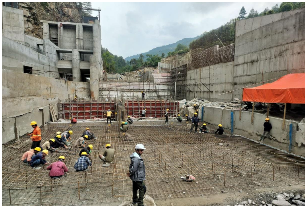
Rebar works at stilling basin
