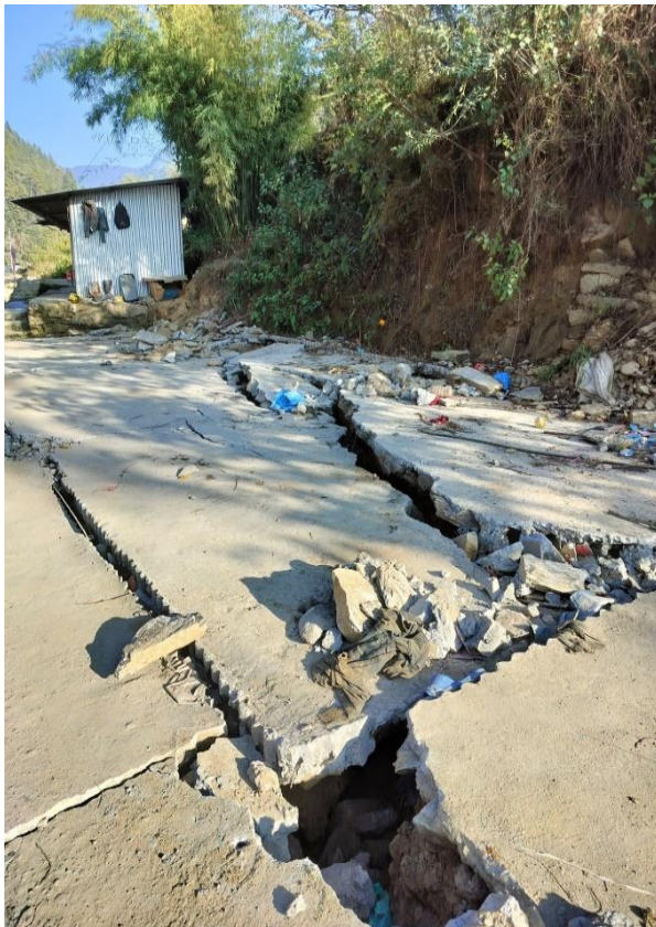
Left Bank Cracks at Headworks
