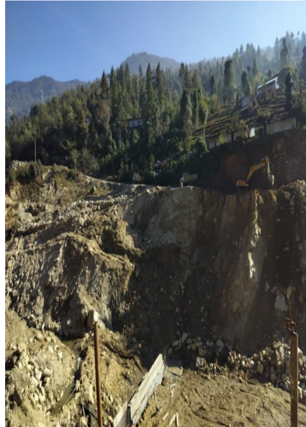
Left Bank Cracks at Headworks
