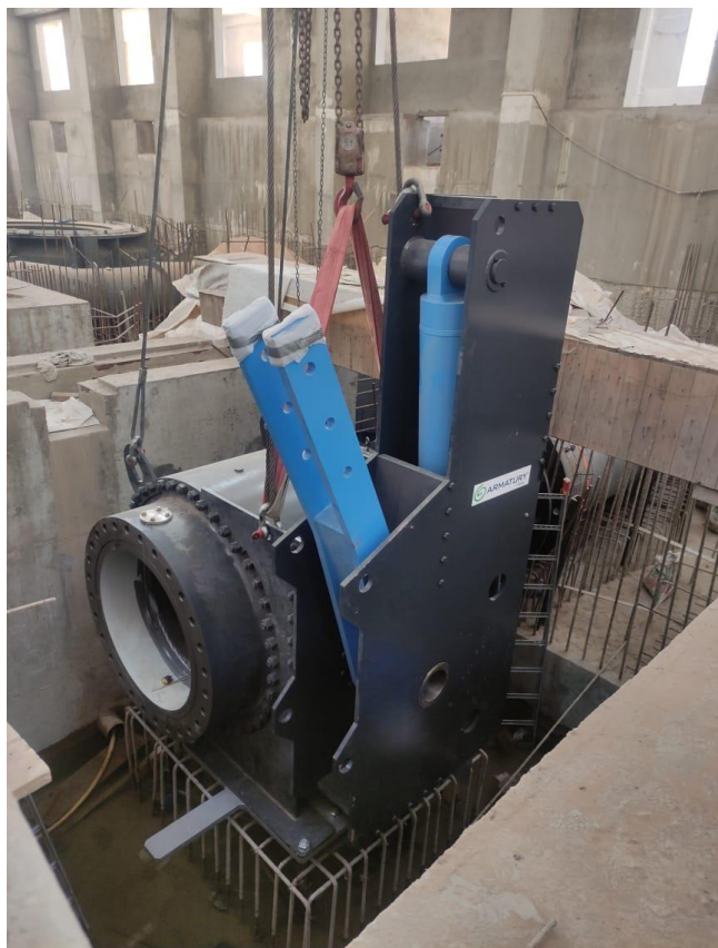
Installation of Unit 3 MIV
