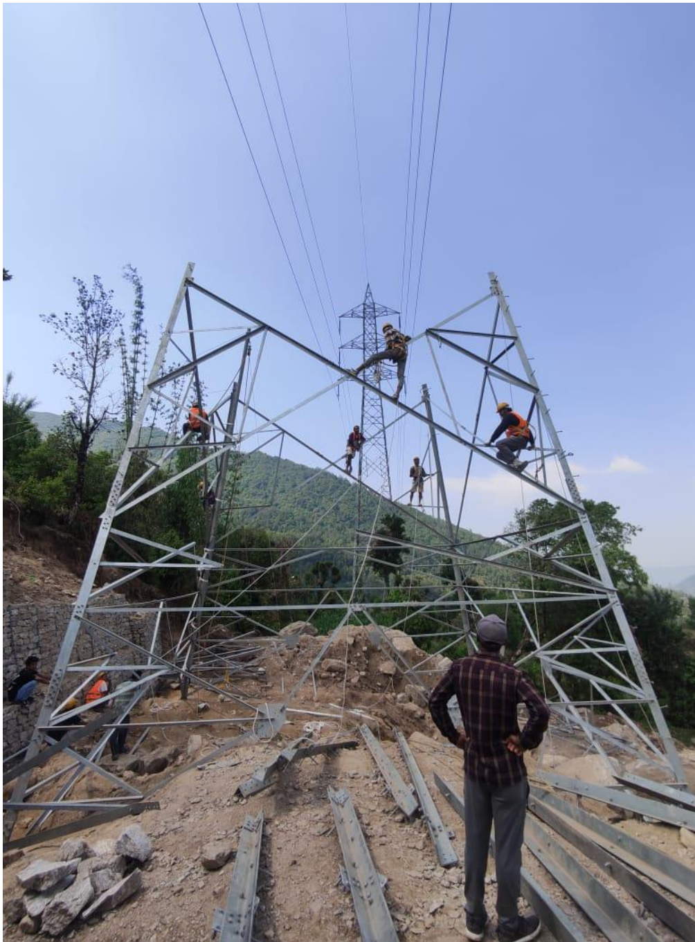
Erection works of dead end tower
