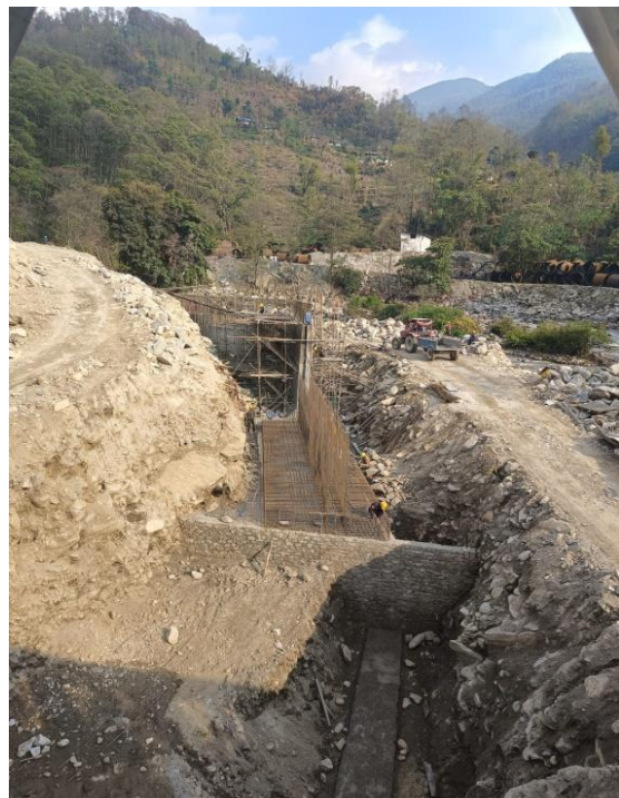
Power House Protection Wall: Floodwall
