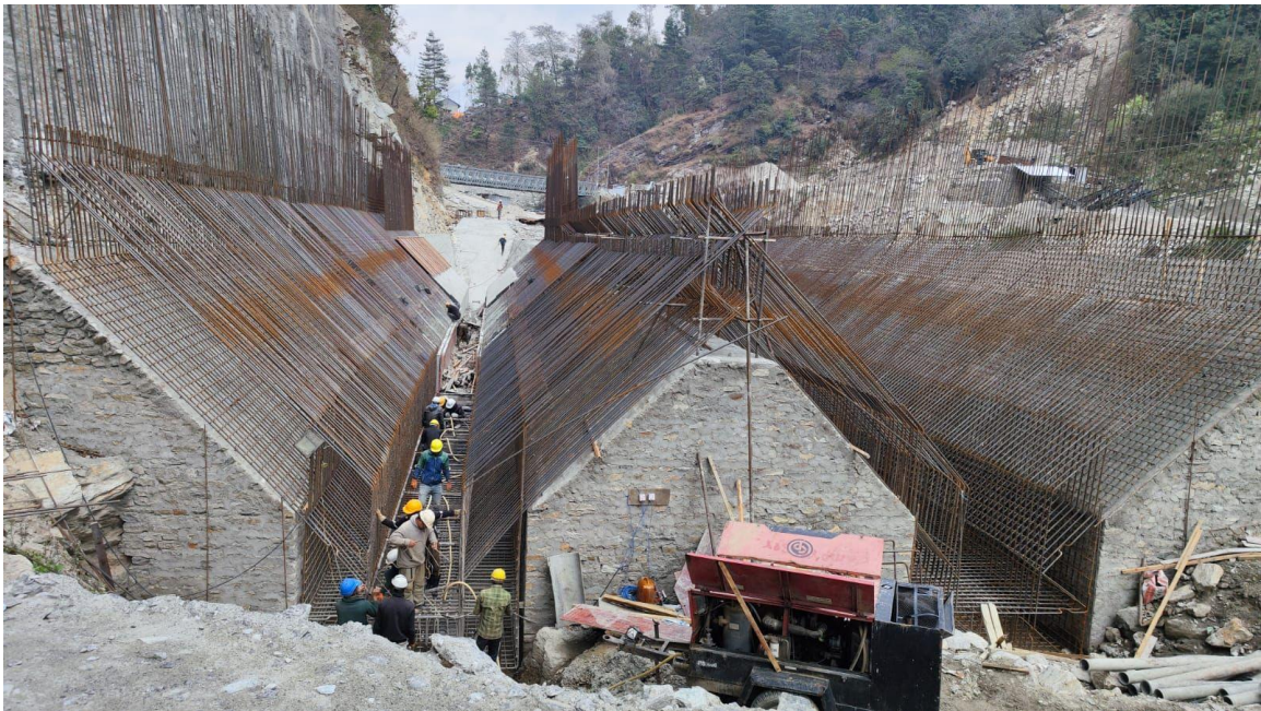
Settling Basin rebar work
