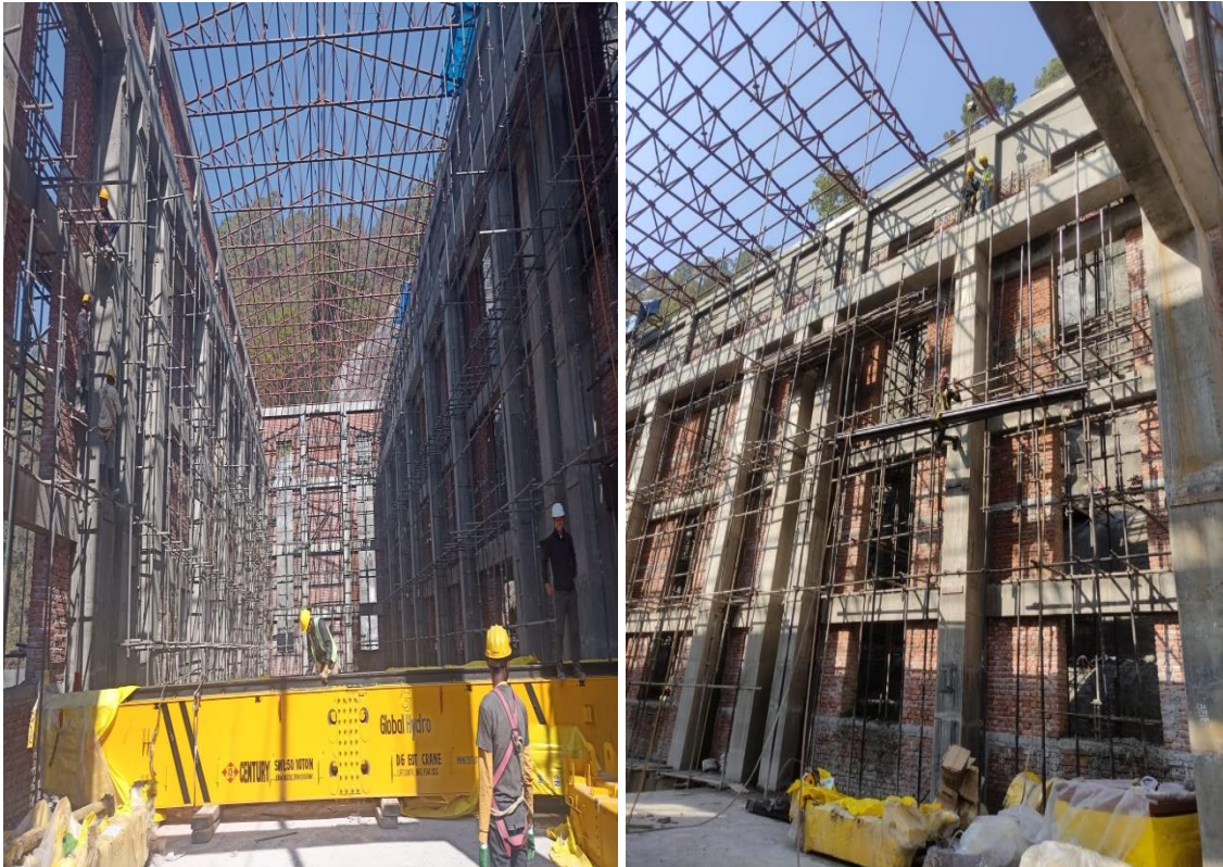
Power house & E.M works (Rail lifting to overhead crane beam)
