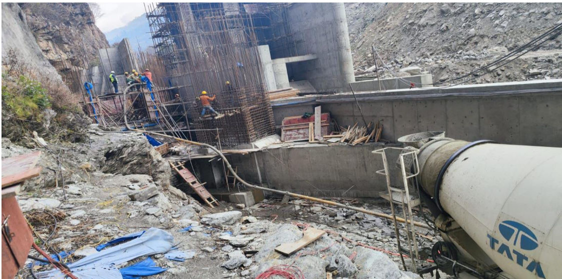
Undersluice panel rebar work
