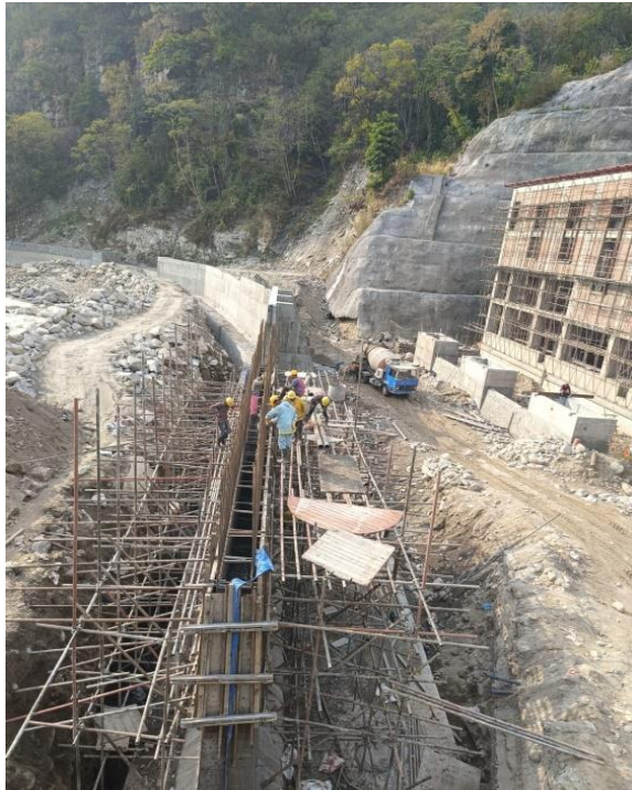
Power House Protection Wall: Floodwall
