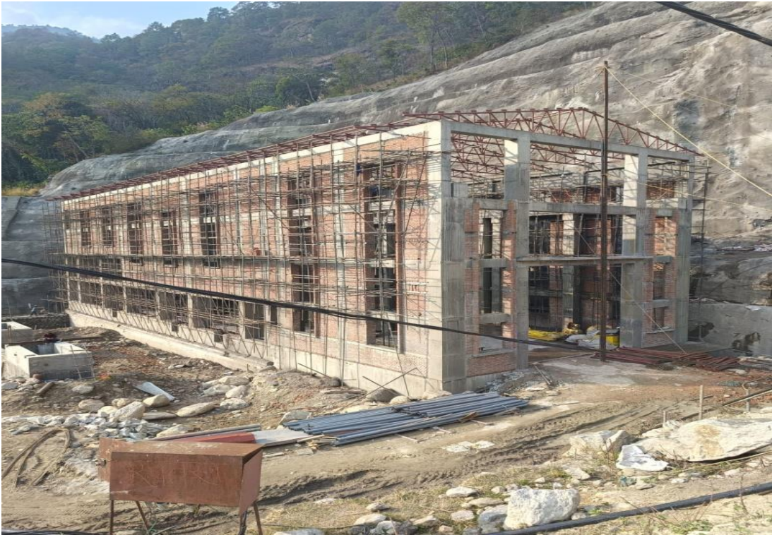
Powerhouse Site Truss Works
