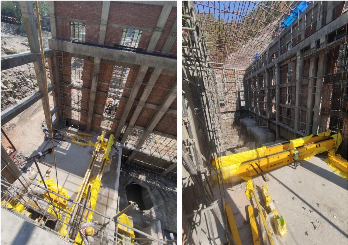
Assembly of EoT crane girders
