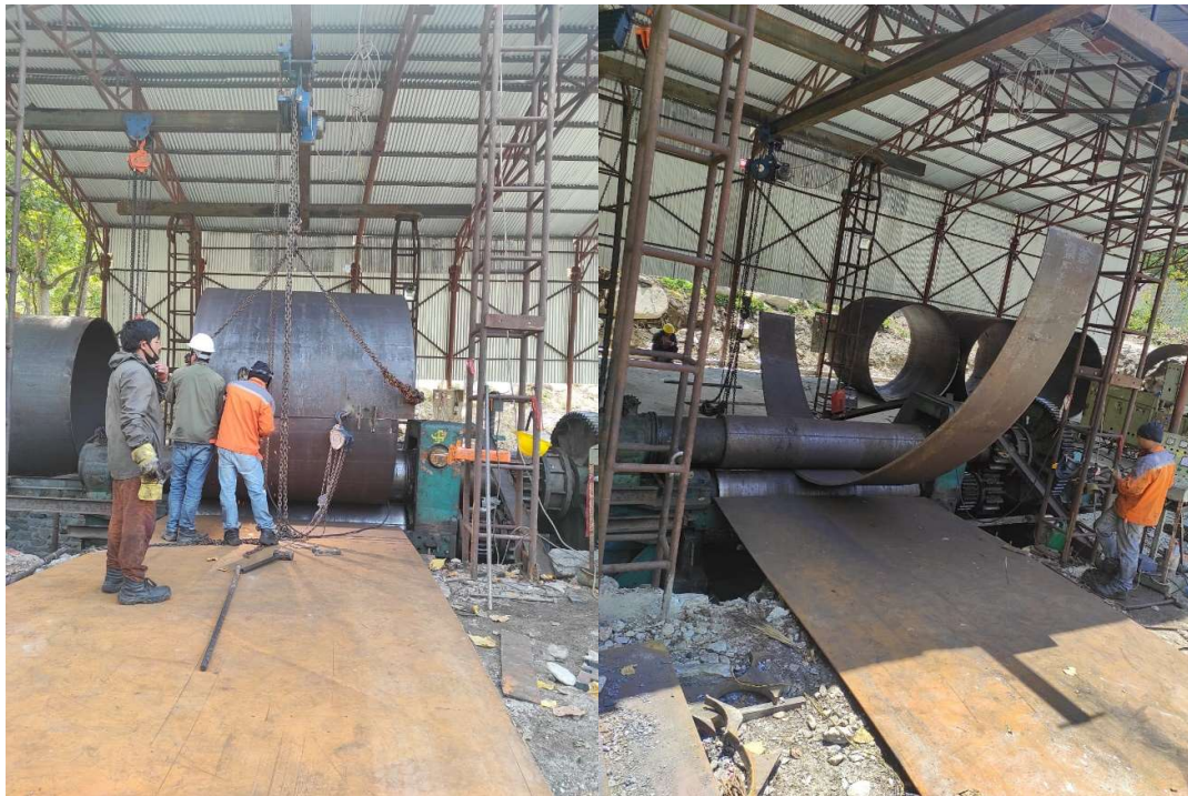
MS- Pipe Rolling operation for Penstock at HM Workshop
