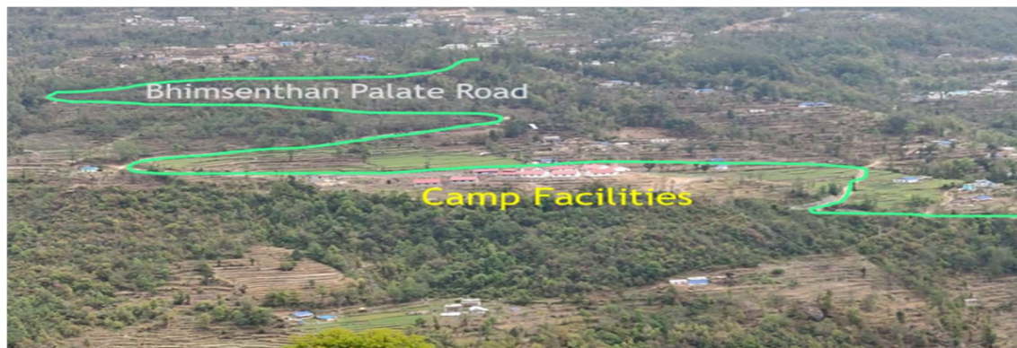
Bhimsenthan-Palate Access Road
