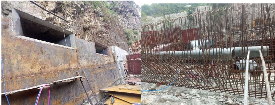
Steel lining works at Bellmouth area- Intake site
