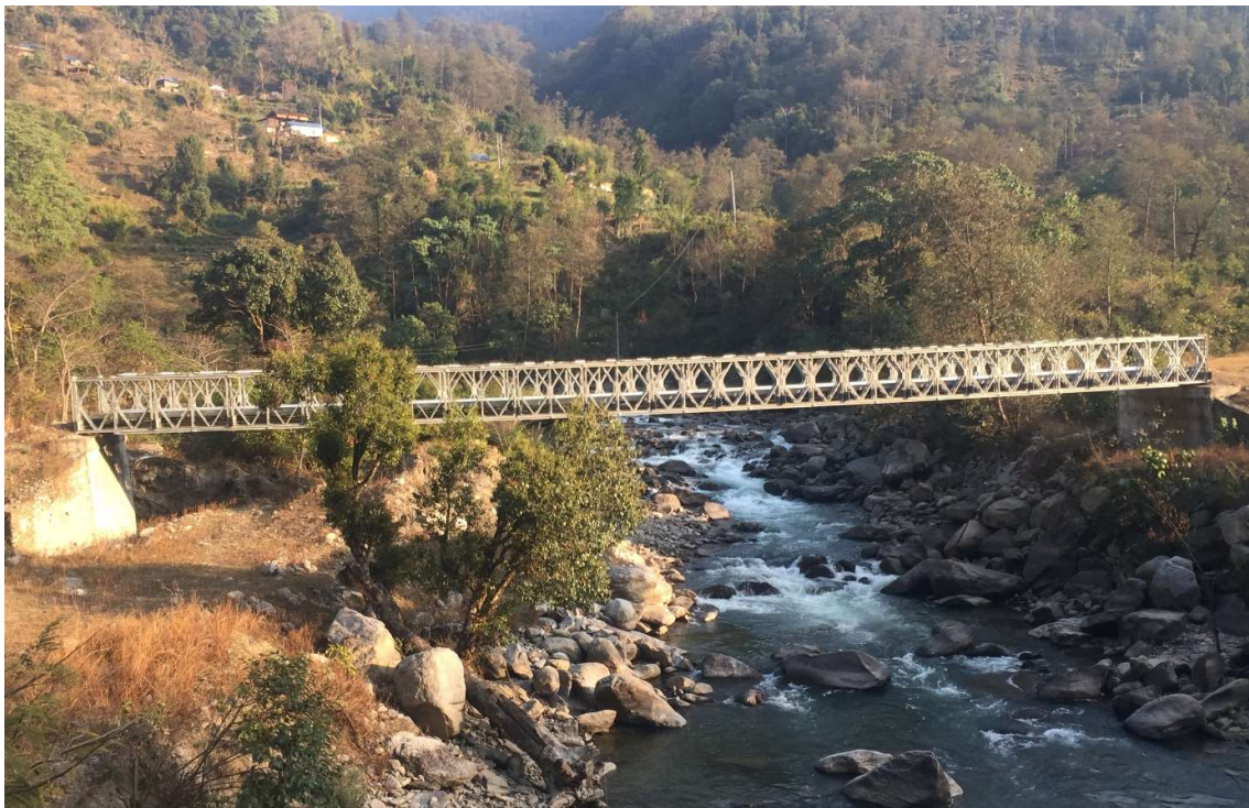
Bailey Bridge III: Hawa-Palate Bridge
