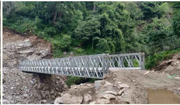
Bailey Bridge II: Hodampa Bridge
